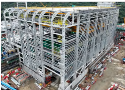
Turbine Building construction
