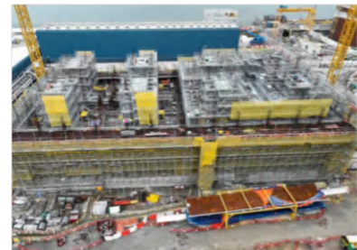
Cooling tower construction
