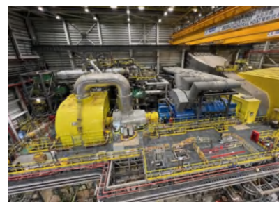
Turbine hall overview
