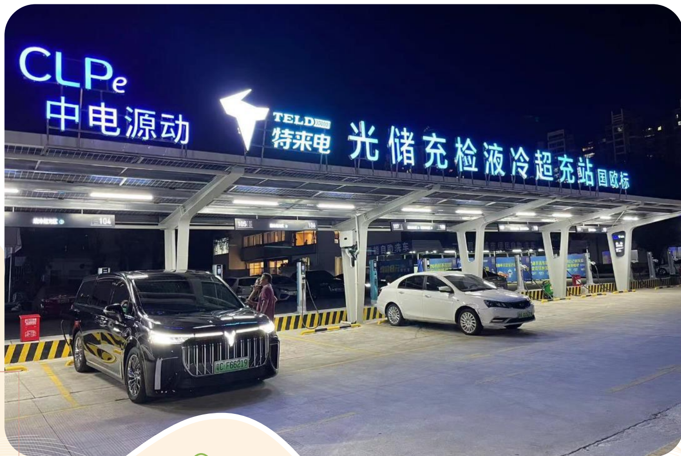
Super-fast Charging Station in Zhuhai, Mainland China.
