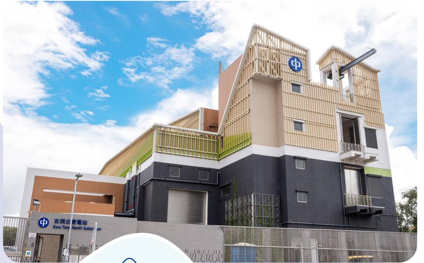
Kwu Tung North Substation, Northern Metropolis, Hong Kong.
