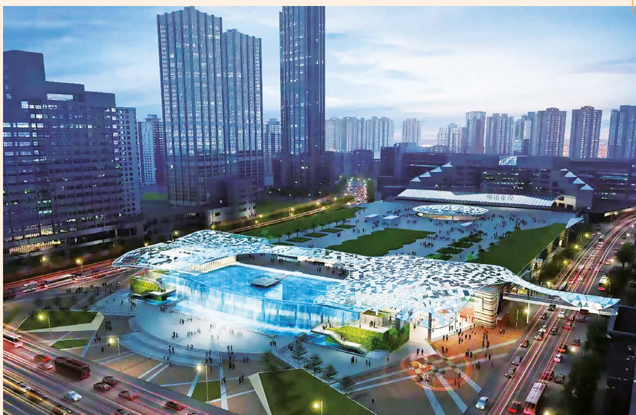
CLP began a comprehensive upgrade of the centralised cooling system at Po Park Shopping Plaza in Guangzhou in 2021 and will operate the retail complex's cooling services until 2036.
