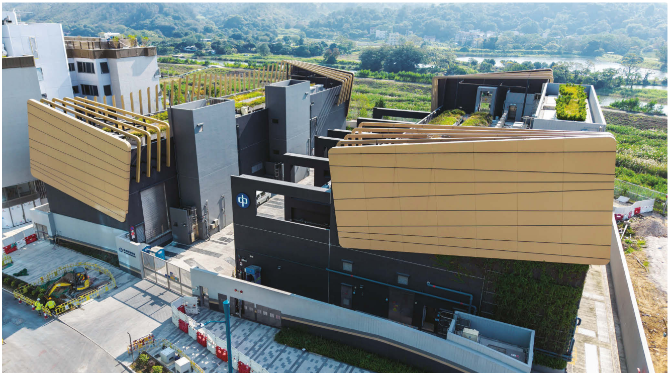
In support of Hong Kong's long-term growth, CLP Power has commissioned three substations in the Northern Metropolis, including the Ho To West substation pictured here, to meet the region's electricity demand.
