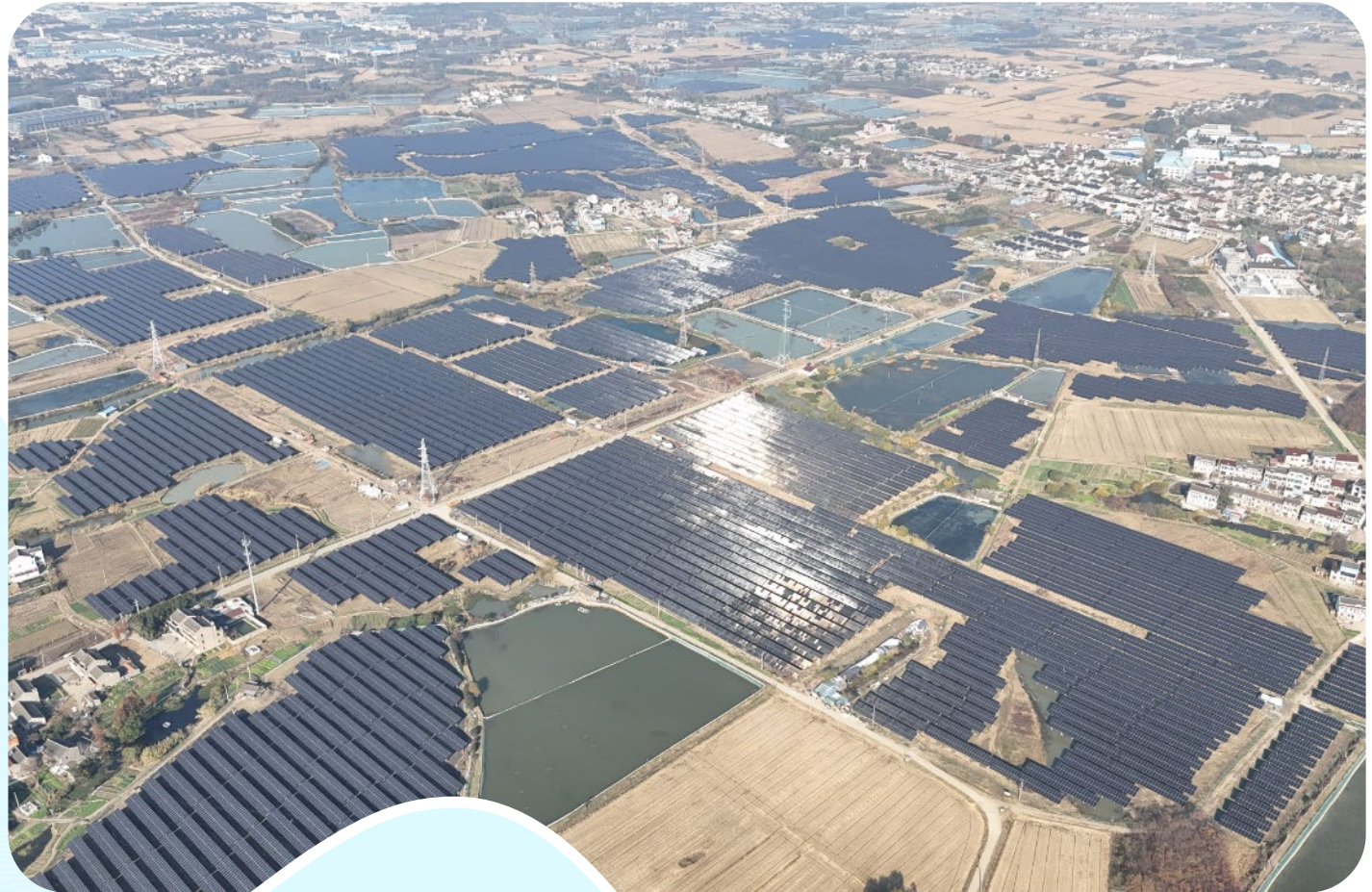
Yixing solar located in Jiangsu Province, Mainland China.
