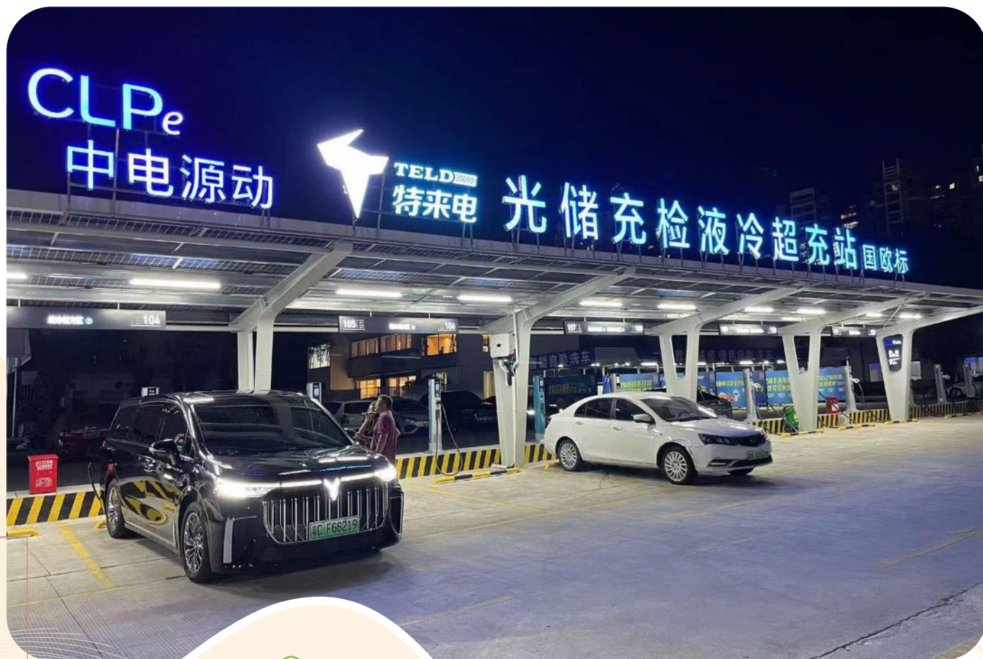
Super-fast Charging Station in Zhuhai, Mainland China.
