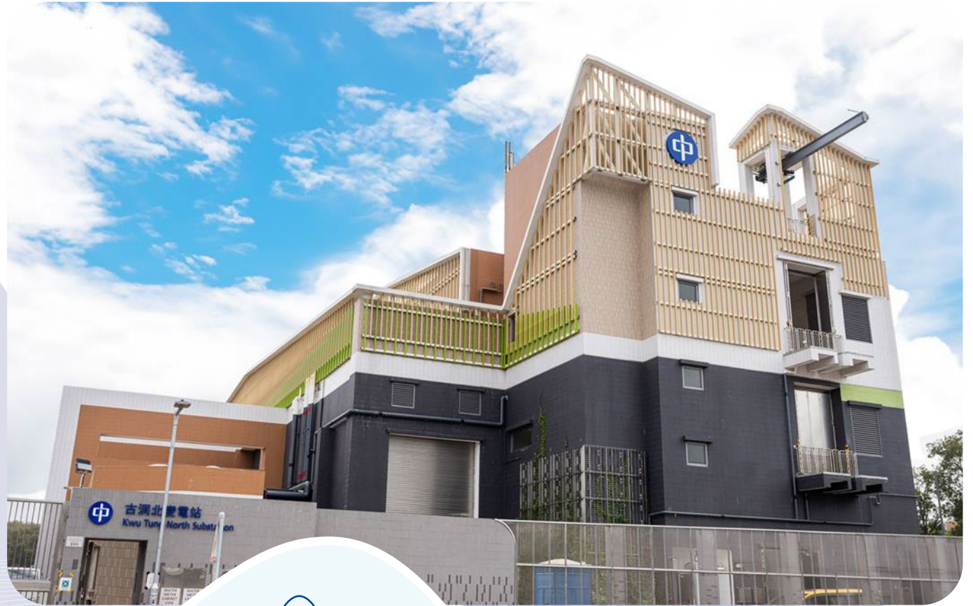
Kwu Tung North Substation, Northern Metropolis, Hong Kong.
