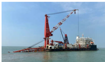
Subsea pipelaying works completed
