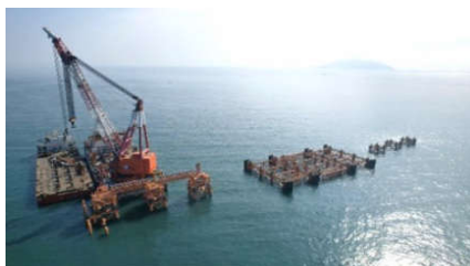
All jackets installation completed
