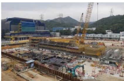
Completed turbine building foundation
