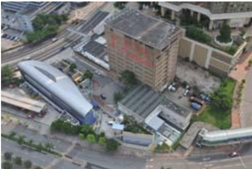
Featured on the right is the aerial view of CLP Sky Woodland while the building on the left is the CLP Sham Mong Road Substation.
