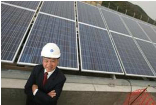
Poly Crystalline Silicon technology is adopted for the Town Island Renewable Energy Supply Project. Featured in the photo is Mr Paul Poon, Director, Power Systems of CLP Power.
