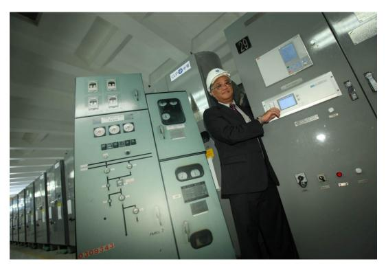
Mr. Ng Wah On, Senior Project Manager (East) of CLP Power introduces the latest 132kV Smart Switchgear (his left hand side) installed in Eastern Road Substation. The switchgear equips with Intelligent, Protection, Automation, Control and Supervision System, which enables more accurate online condition monitoring. Featured on his right hand side is traditional 132kV switchgear.
