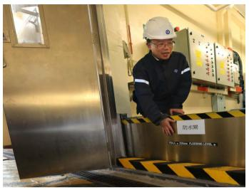
CLP Power Chief Operation Officer Chow Tang Fai demonstrates the installation of a flood gate at the entrance of a transmission substation.
