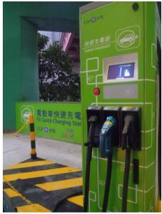
New multi-standard quick charger at Sheung Tak Estate in Tseung Kwan O can charge most EVs up to 80% within 30 minutes, providing enough power for a journey of approximately 100 km.
