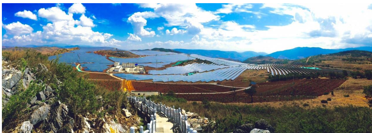
The 50MW Direct Current capacity Xicun I Solar Power Station occupies a site of 86 hectares with a total of 204,600 solar panels installed (click here for a video on the project).
