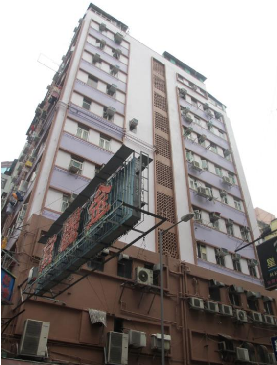
Subsidised by CLP Eco Building Fund, Cheung Hing House in Mongkok has replaced its lift motor with a Variable-Voltage-Variable-Frequency control system, saving 30 per cent in the building's annual electricity cost.
