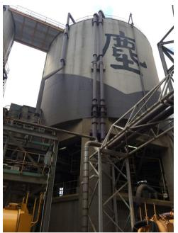
The outlook of a dust storage facility in Castle Peak Power Station: During the process of coal-fired power generation, dust is produced from coal burning. After electrostatic filtering, the dust is collected in the dust storage facilities.
