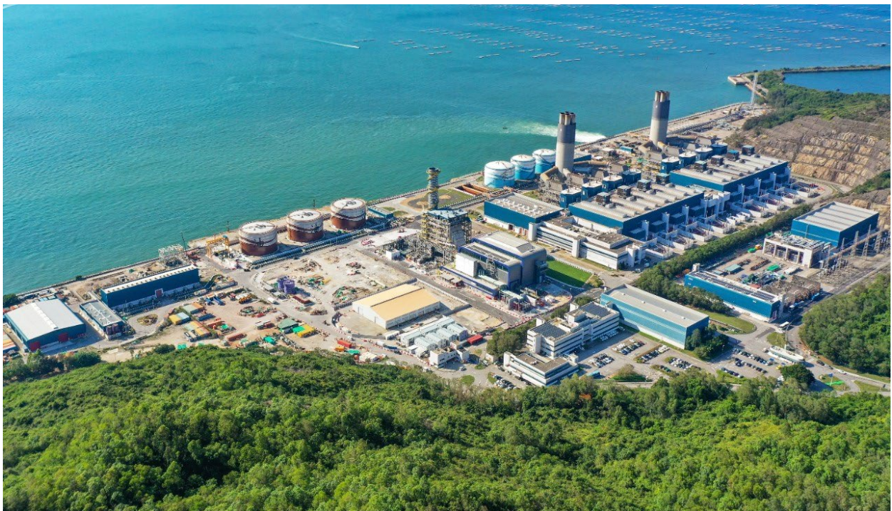
Black Point Power Station is one of the world’s largest combined cycle gas-fired power stations. Eight of its generating units are powered by GE.
