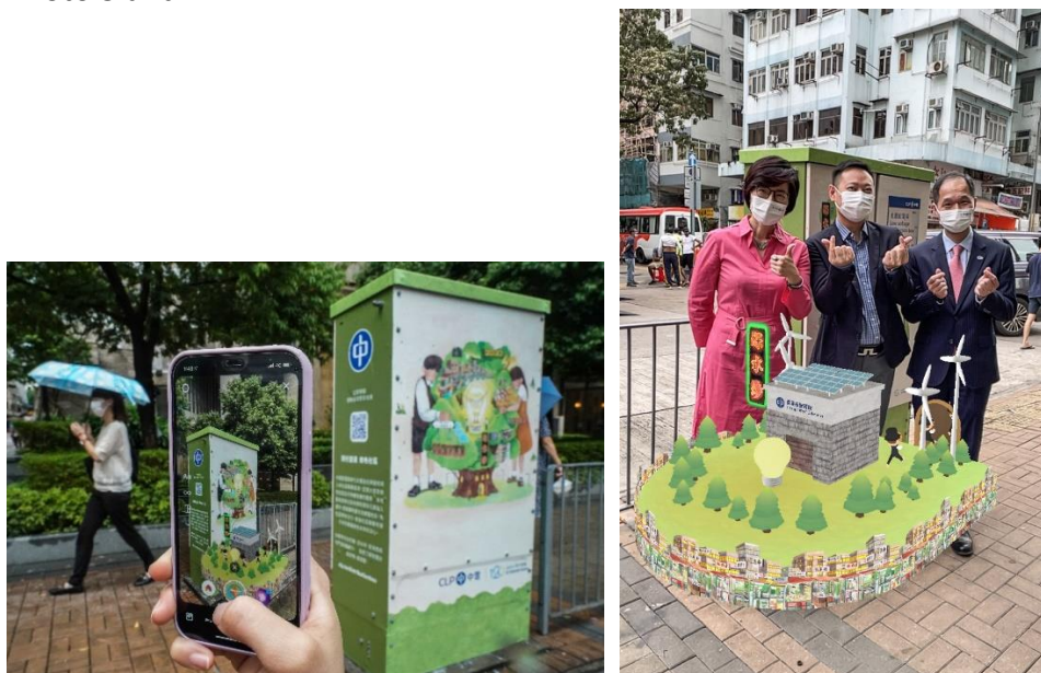
The Distribution Box Beautification Project includes an element of augmented reality to combine art and technology. People can access Instagram features by using their smart phones to scan QR codes on the boxes. (Photo 4 from left) Chief Corporate Development Officer of CLP Power Ms Quince Chong, Secretary for Home Affairs Mr Caspar Tsui and Managing Director of CLP Power Mr T K Chiang took selfies with the special filter.
