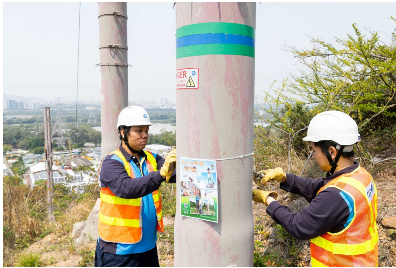
Safety warnings are displayed at CLP Power's transmission poles to remind citizens to prevent hill fires.
