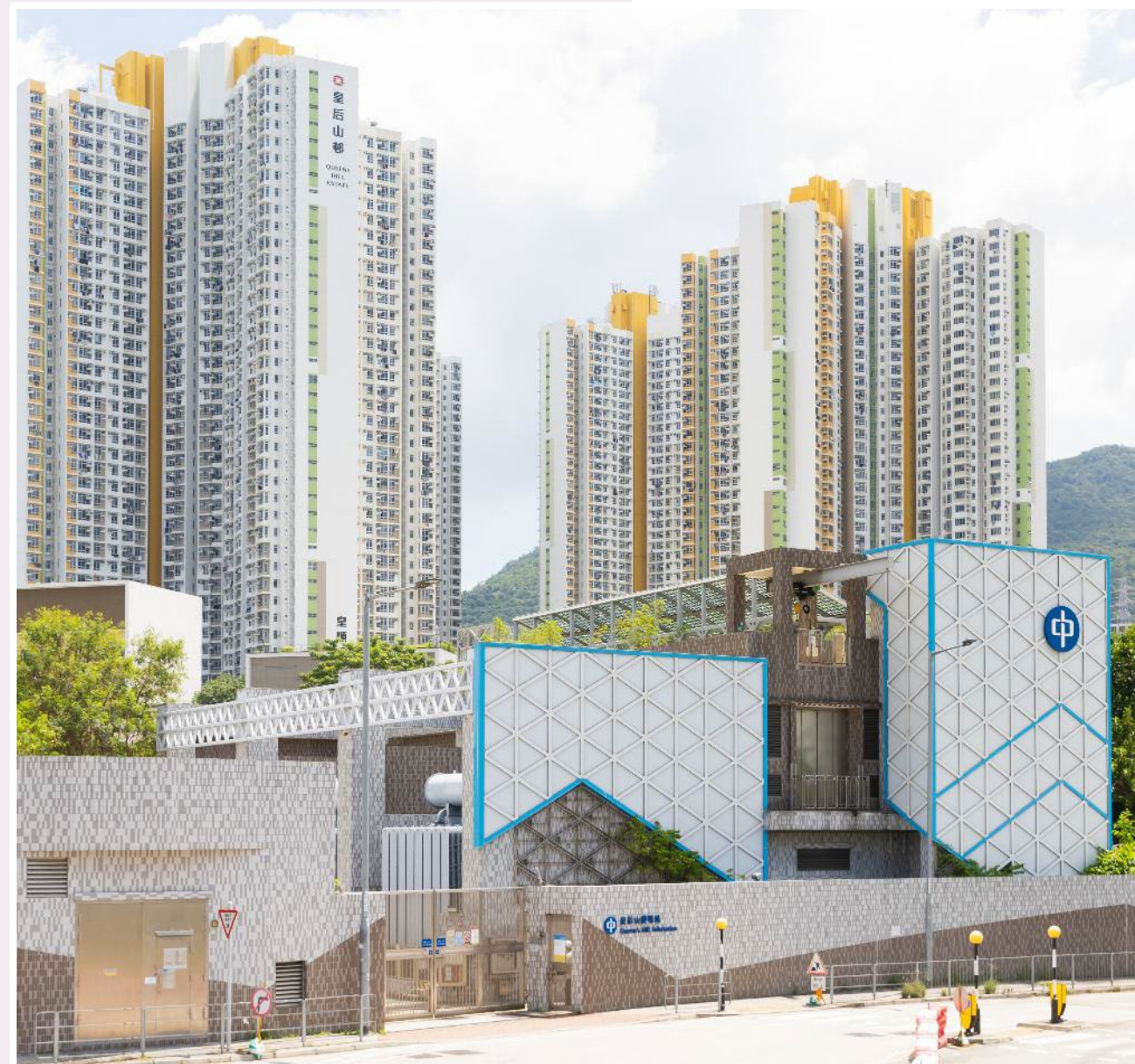
Queen's Hill substation in Fanling, Northern Metropolis, Hong Kong.
