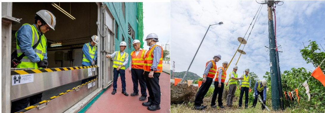
Mr Poon Kwok Ying, the Director of Electrical and Mechanical Services is briefed on CLP Power's forward-looking preparations in response to extreme weather, including flood protection measures at substations and maintenance works on overhead lines.
