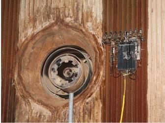
"Our boiler is as tall as a 30-storey building," says Kelvin Sa, a member of the boiler inspection team. "With the robot that can crawl up the boiler wall in no time like 'Spider Man', we can significantly reduce the use of manpower which means a great improvement in safety."
