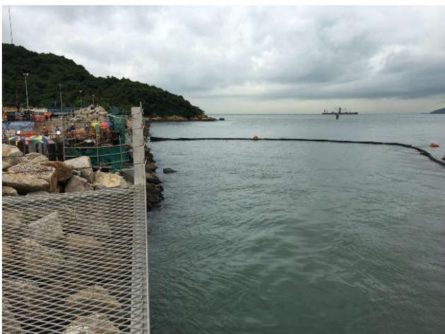
Use of silt curtain as precautionary measure to prevent construction works near the sea from causing suspended sediment impacts to marine environment
