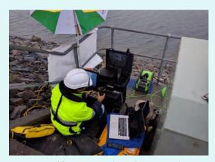
ROVs are used for inspecting the cooling water inlet tower in the Mount Piper thermal plant in Australia.
