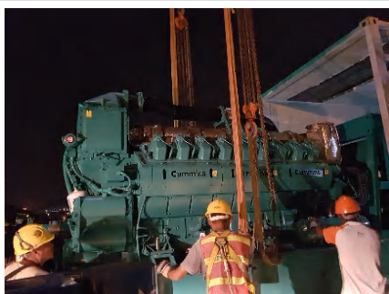
Delivery of generator sets
