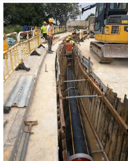
Gas pipeline laying along Nim Wan Road
