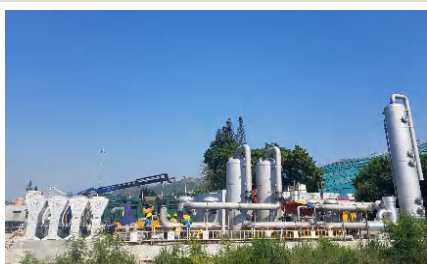
Delivery of gas pre-treatment system equipment
