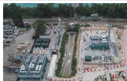
An overview of the project site
